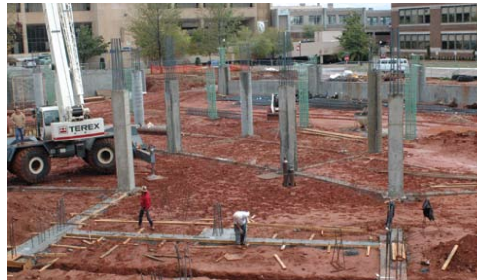
Construction progress on new DMEI facilities
