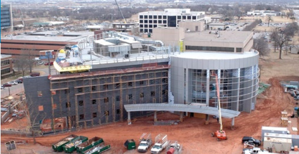
Construction of building expansion.
